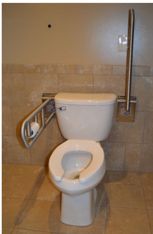
View of accessible shower (left) and toilet with movable handicaps bars on both sides to help residents with cares and lifts as needed (right)
