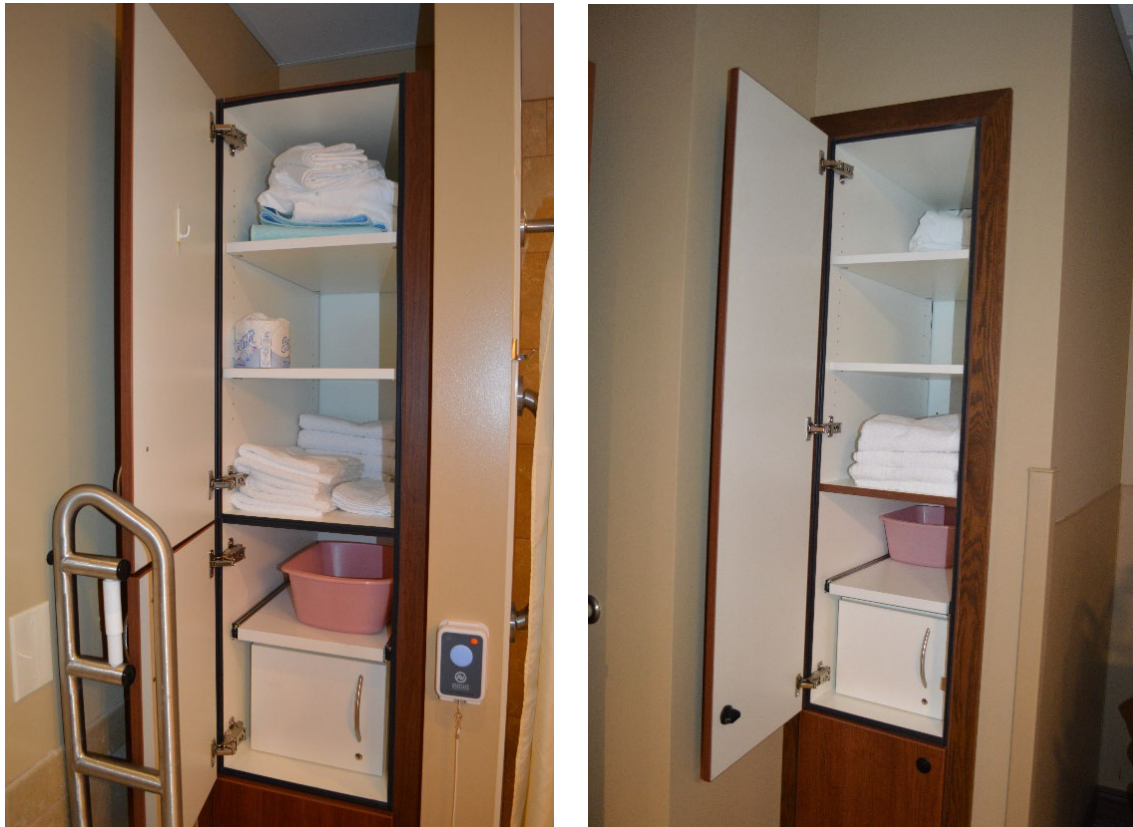
The same nursing server cabinet open from inside the resident's room (left) and through hallway (right). Allows restocking of supplies and towels without disturbing resident.
